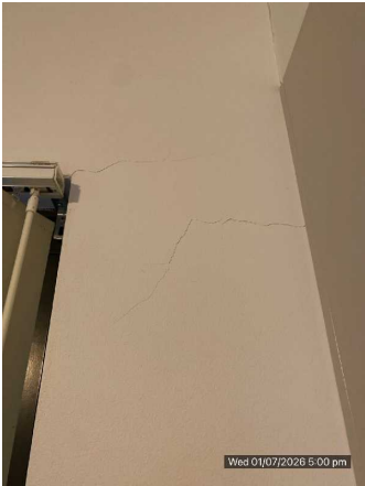
Studio: Walls/picture hooks (photo 1 of 1)
