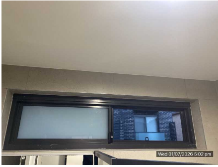
Bathroom: Windows/screens/window safety devices (photo 1 of 1)
