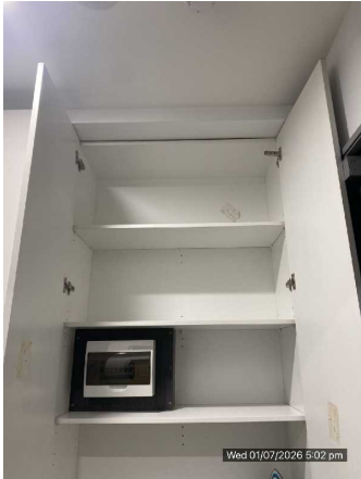
Entrance/Hall: Storage (photo 3 of 3)
